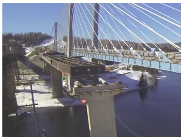
Here the old Nipigon bridge (on left) has been rolled past the first pier towards disassembly on the far shore.
