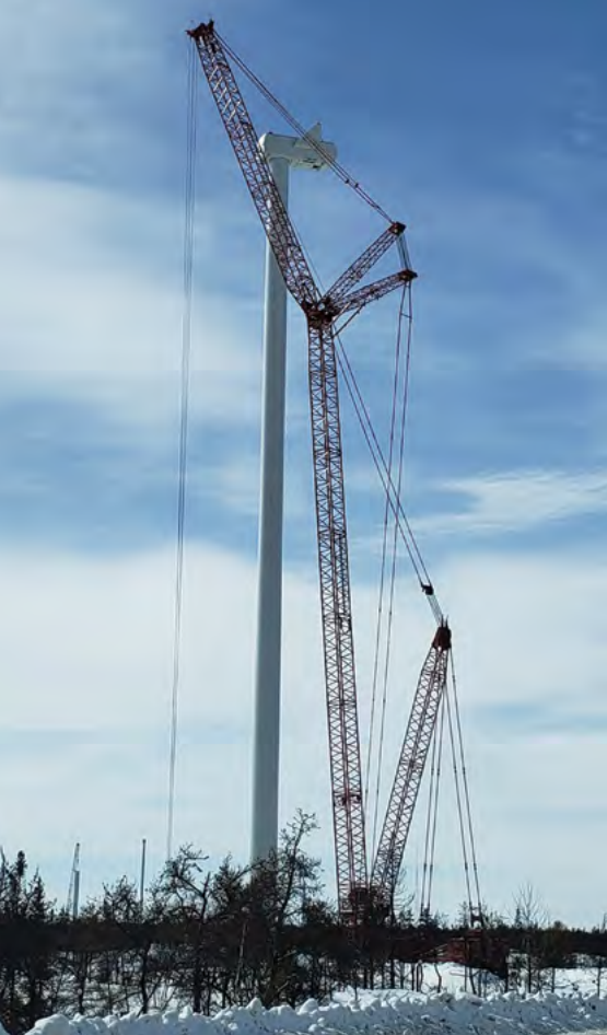
Prep For Hub Install. Photo courtesy of Patten Energy.
