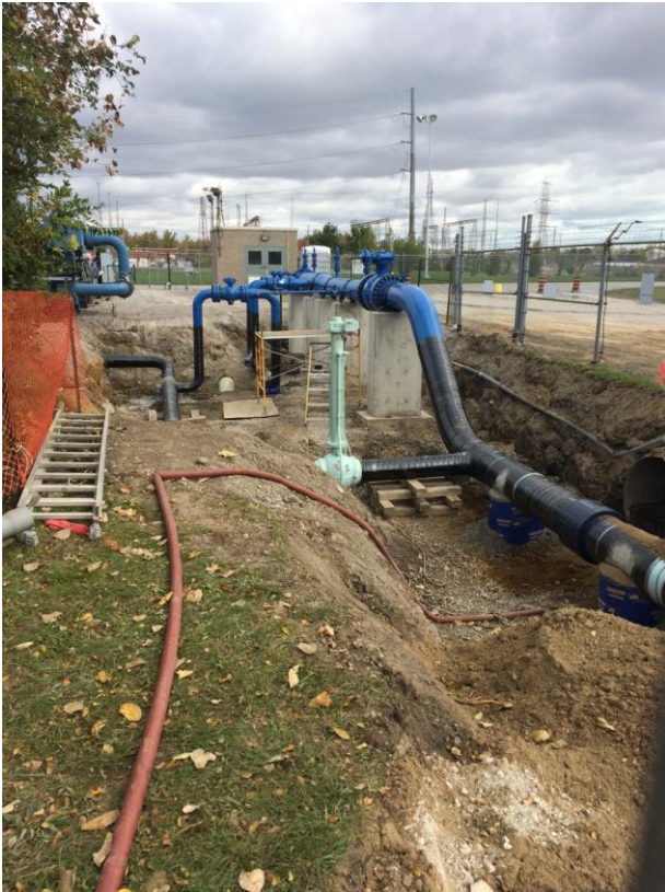
Gas pipelines relocated
