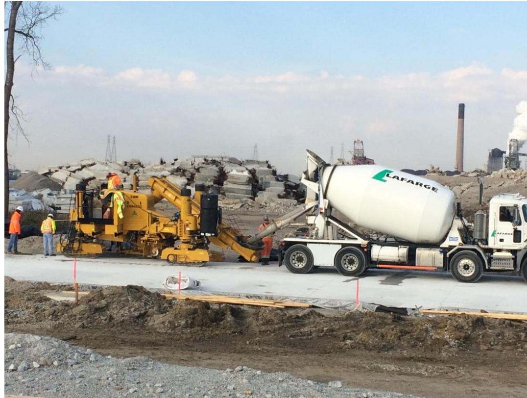
Perimeter access road.
