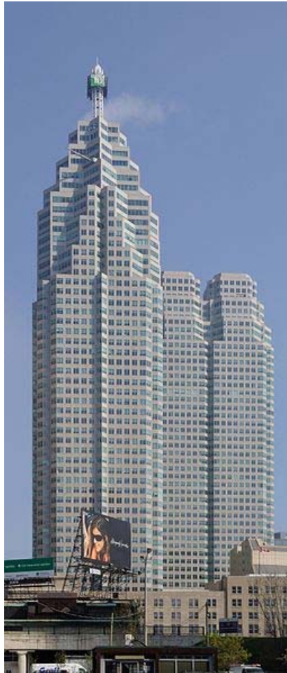
TD Canada Trust Tower , the tallest building completed in Toronto in the 1990s
